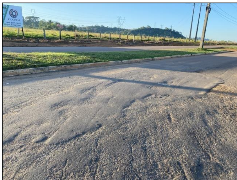
Figura 24 – Remendos Trecho A (a)
